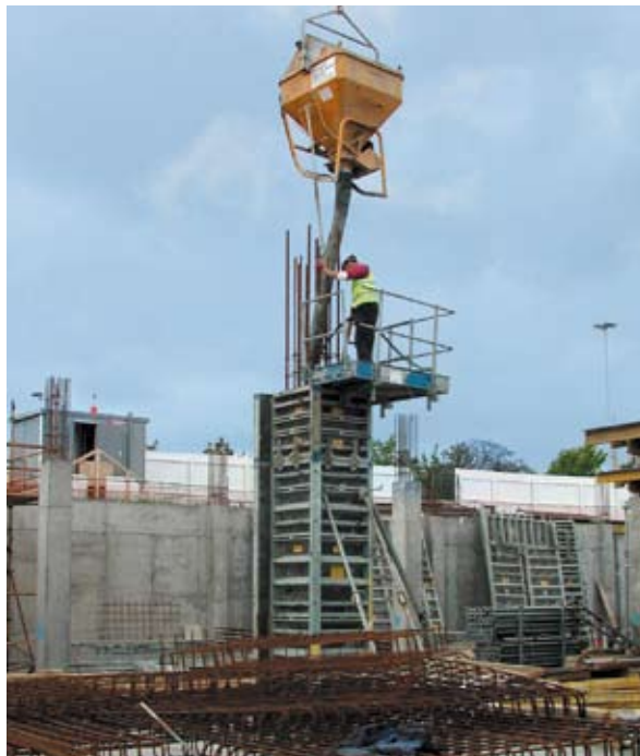
System column formwork, shopping centre, Telford, Shropshire (courtesy Doka)
