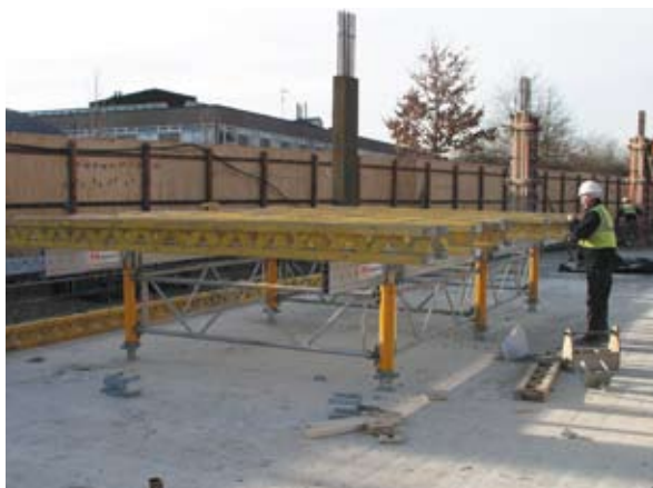
Ground level assembly of table forms (courtesy Peri)
