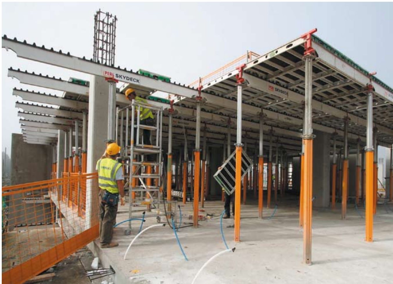
Modular system formwork (courtesy Peri)
