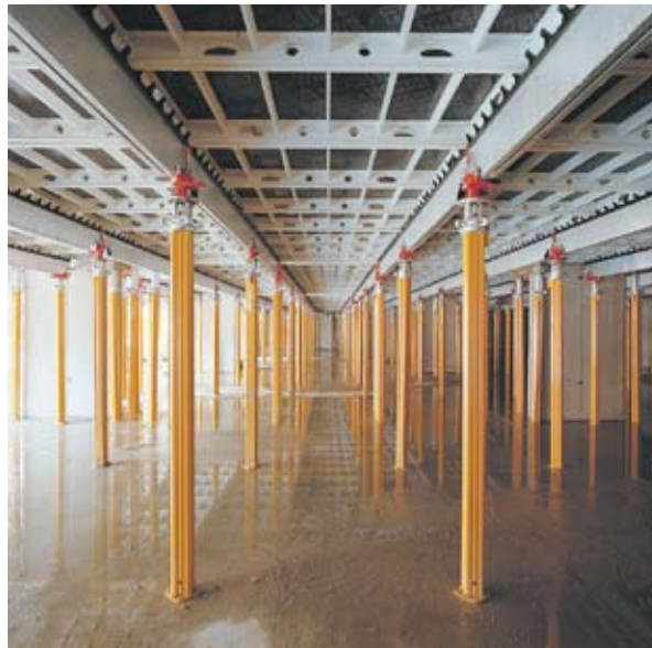
Structural finishes and modular system formwork (courtesy Peri)
