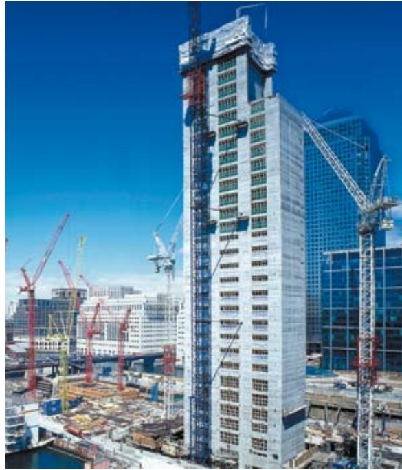
Slipformed core of HQ3, Canary Wharf, London (courtesy PC Harrington)
