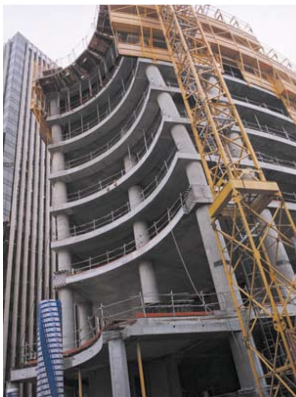
Inclined circular column formwork, PC6 Tower, Paris (courtesy Outinord/G Hendoux)
