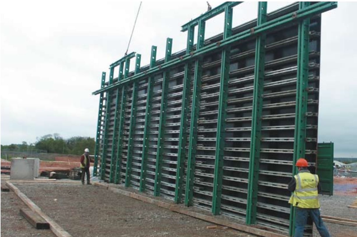
Wall formwork, RAF Museum, Cosford, Staffordshire (courtesy A-Plant Acrow)
