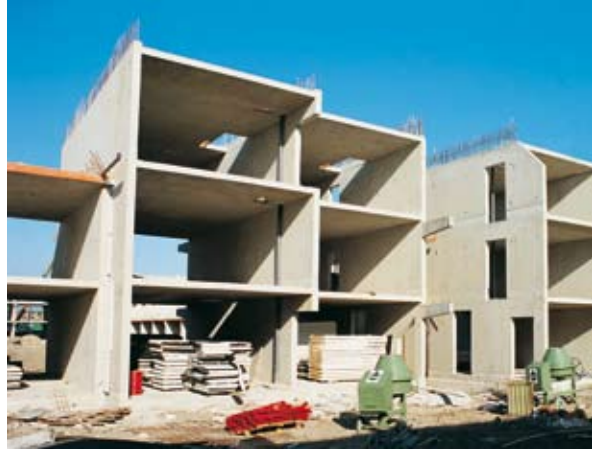
Residential tunnel form structure (courtesy Outinord/G Hendoux)
