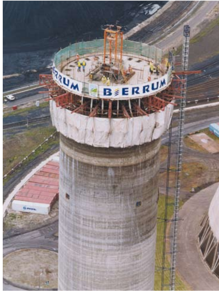
Slip-formed 200m chimney at West Burton power station, Nottinghamshire (courtesy Bierrum)
