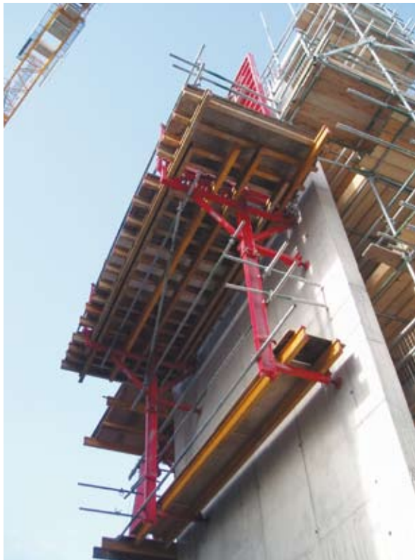
(Courtesy A-Plant Acrow)
