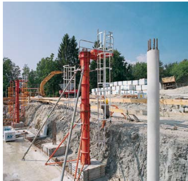
System column formwork (courtesy Peri)
