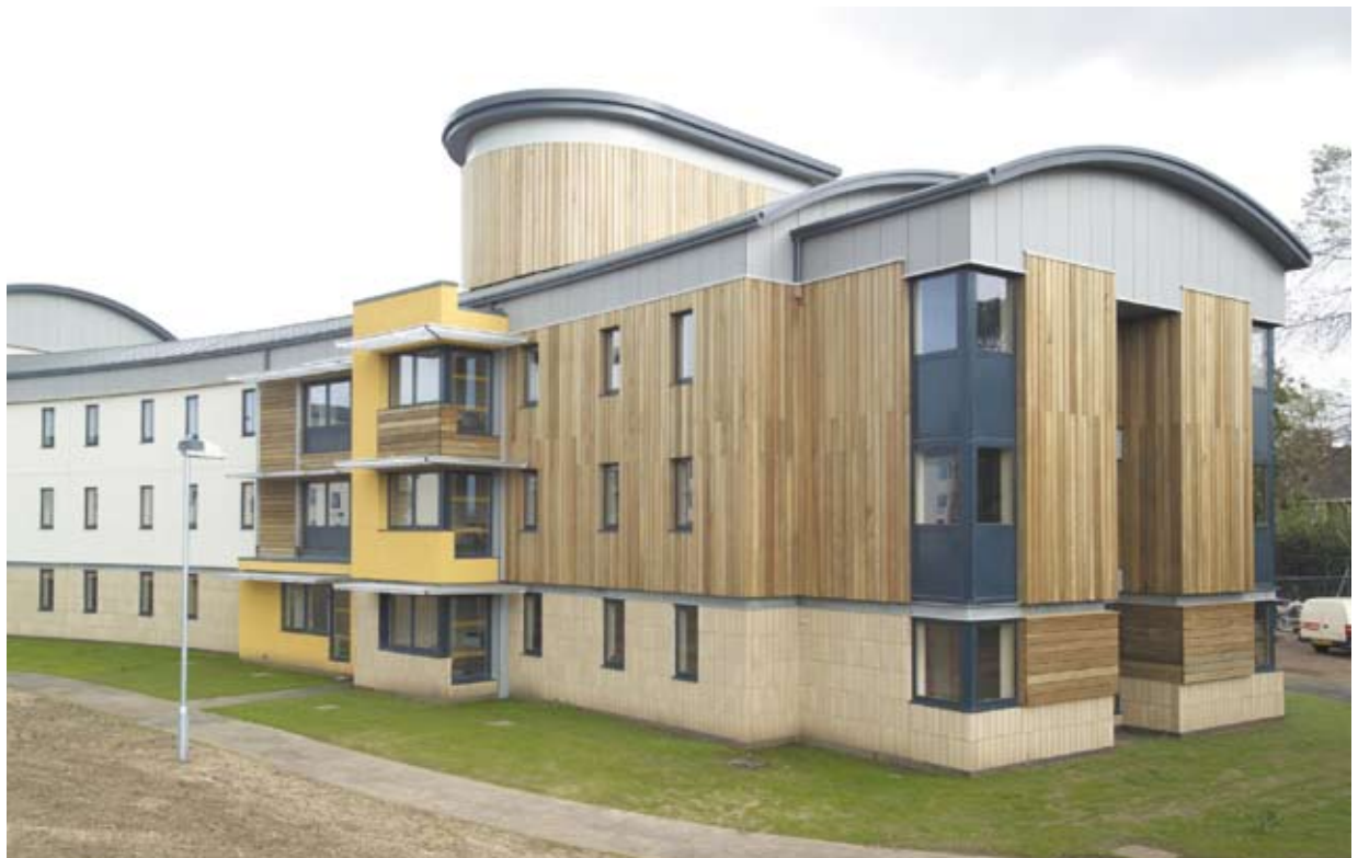
Student accommodation at University of East Anglia – tunnel form structure (courtesy The Concrete Centre)
