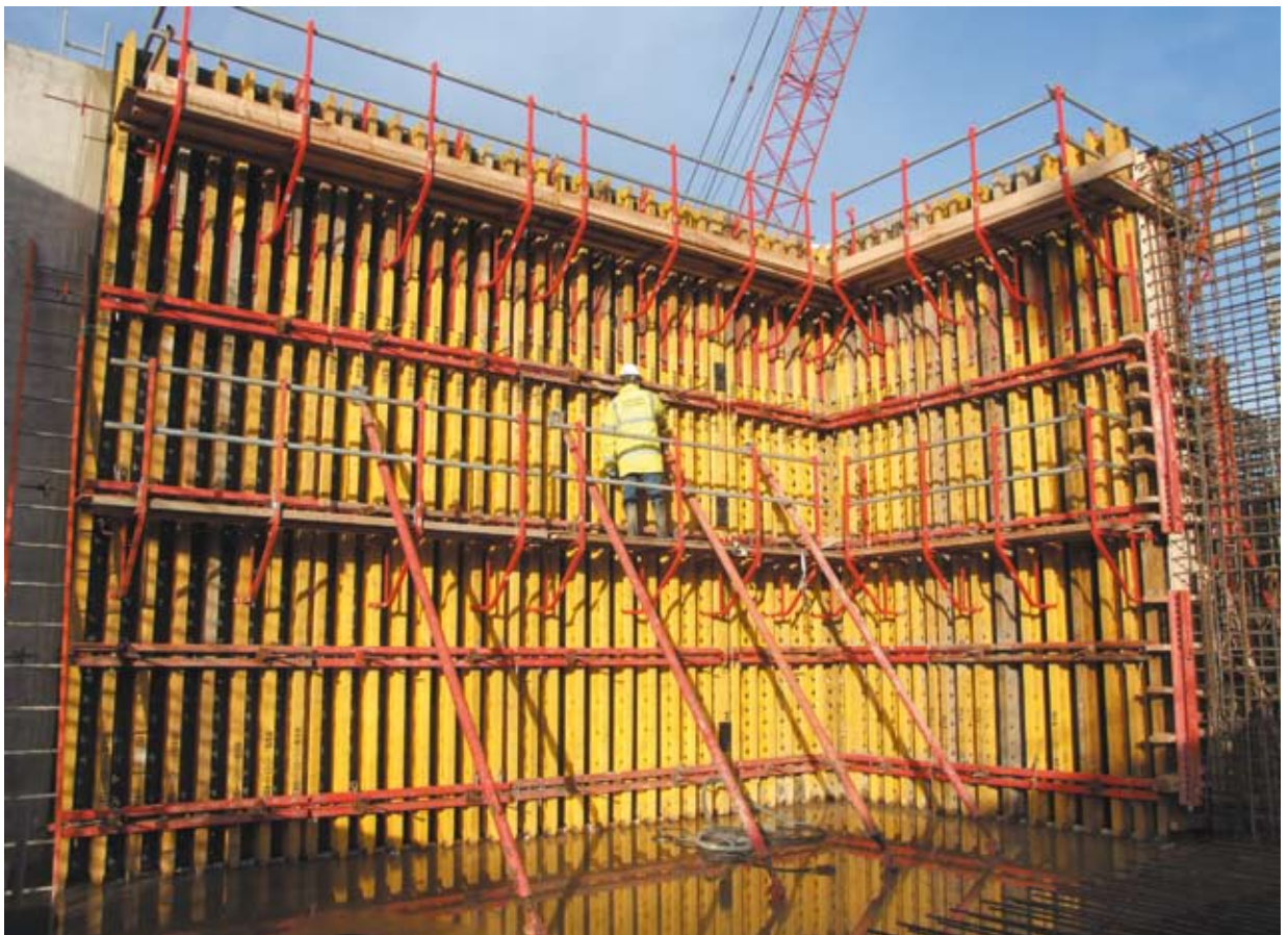
System wall formwork (courtesy Peri)
