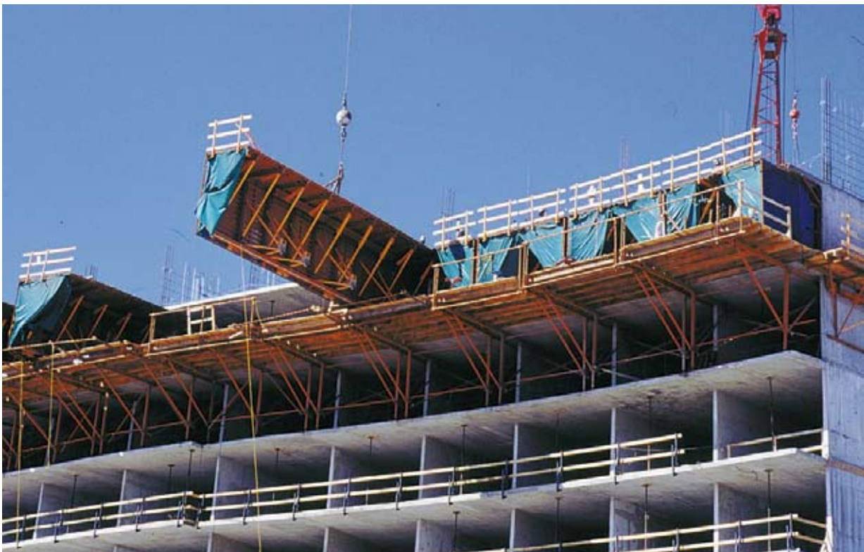
Tunnel form structure – hotel in Lucaya, Bahamas (courtesy Outinord/G Hendoux)
