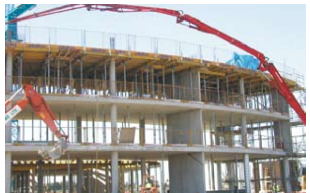
Secondary school, Solihull, Birmingham using table forms (courtesy Doka)
