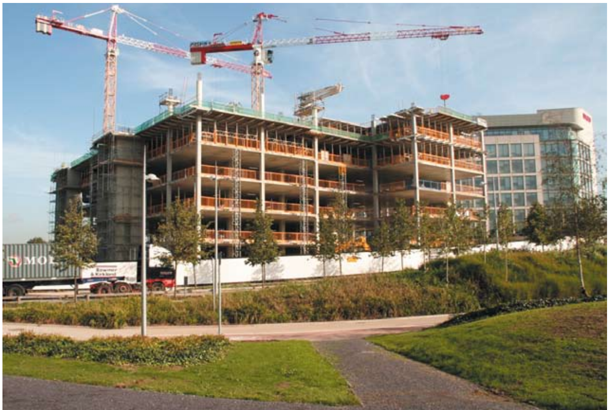
Office development, Park Royal, London – lightweight aluminium formwork systems (courtesy Peri)
