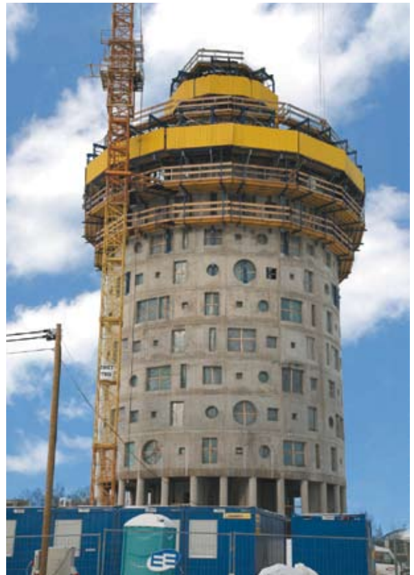
Mixed office/residential development, Tartu, Estonia using self-climbing jump form (courtesy Doka)
