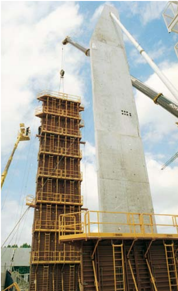
Vertically stacked wallform 22.5m high – Disneyland, Paris (courtesy Outinord/G Hendoux)
