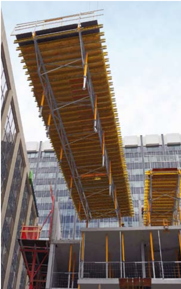
Flying formwork (courtesy Peri)
